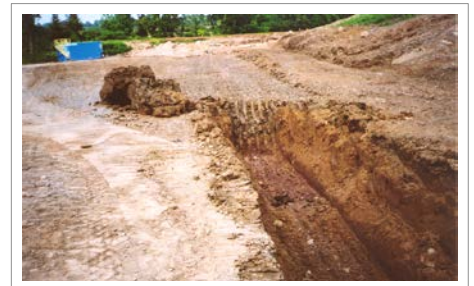
Perimeter Clay Cutoff Wall
